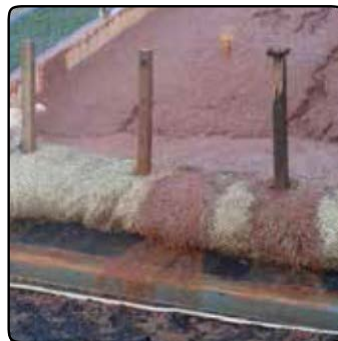
Fig. 6: 20" Straw Wattle (70% Removal Efficiency)
