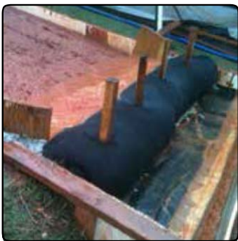
Fig. 2: 12" SiltSoxx™ (97% Removal Efficiency)
